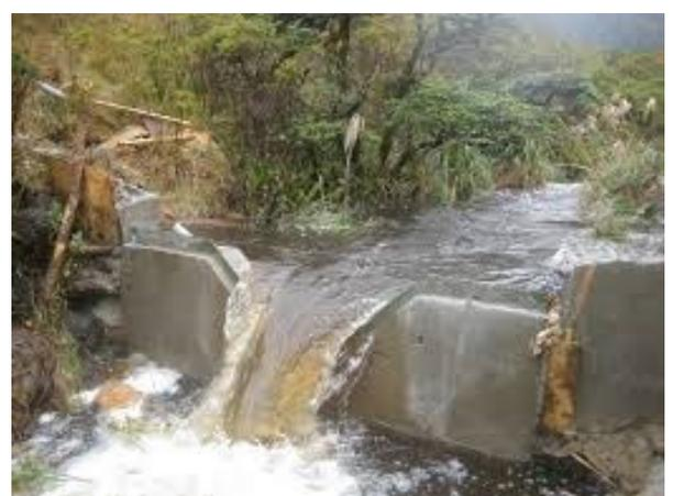
FIGURE 11. (a) A rectangular weir in Kimakia watershed, Kenya. (b) A v-notch weir in Peru. Photos from: Alemseged Tamiru Haile and Buytaert et al. (2014).
