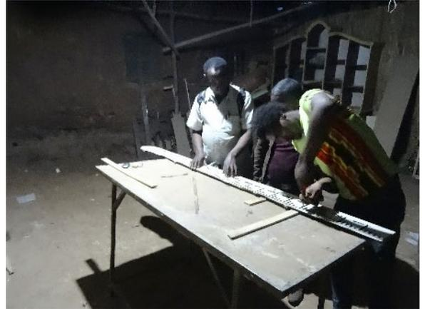
(c) Bolting the wooden planks to the angle iron on the riverbank.
